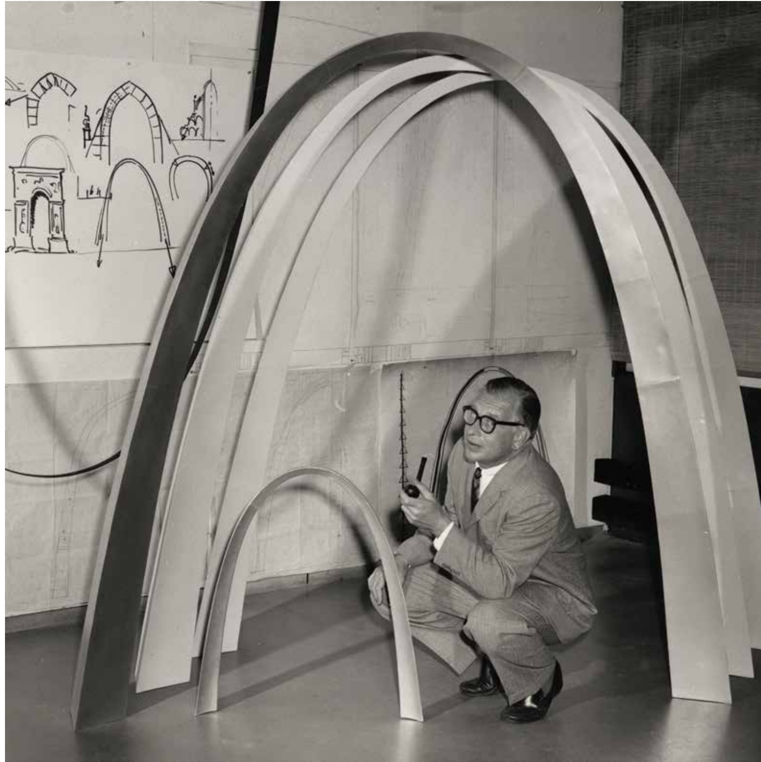
The Gateway Arch in St. Louis. The model of the arch at right has three-edged legs, a suggestion from sculptor Carl Milles (Eero's original idea called for quadrilateral legs). Eero never gave Milles credit for this improvement and Milles packed up and returned to Sweden.
